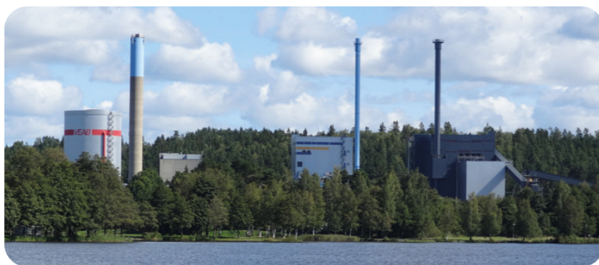
Municipality owned CHP plant. Photo: Växjö Energi AB
