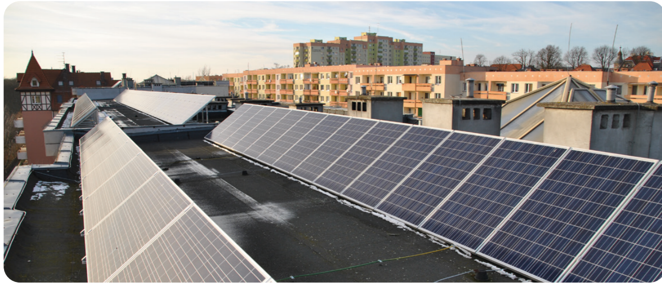
Pszczelna Solar Housing. Photo: Krzysztof Stasiewicz
